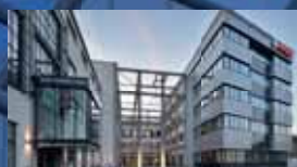
Kotelna park Radlice v Praze
